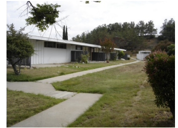
Demolition started this month of Leisure Life Apartments in preparation for a 368 unit Cresta Bella condominium complex. Re-development of the Doubletree is no longer imminent.
